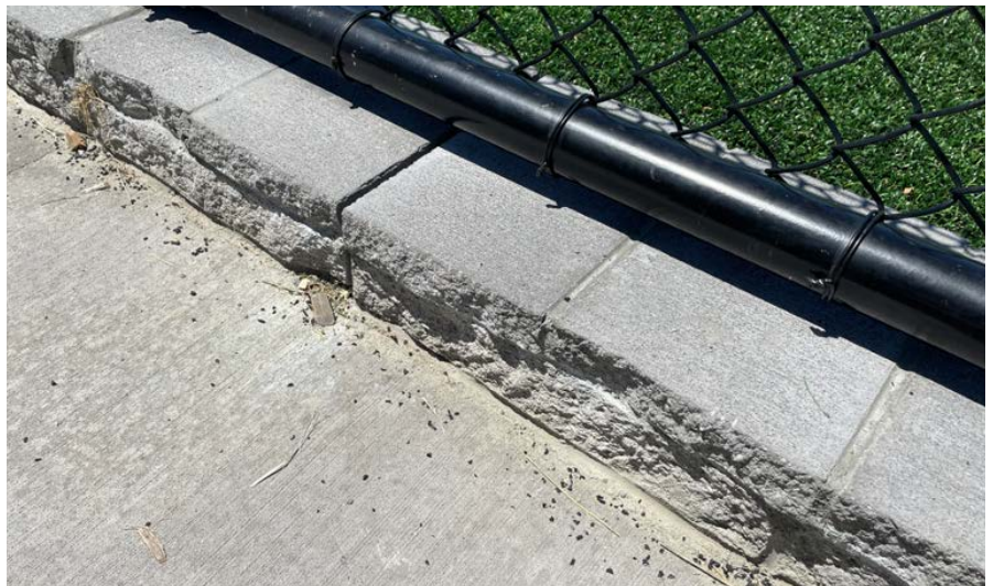
FIGURE 1: An example for tracking of rubber crumb infill from synthetic turf sport fields. The image was taken on 22 February 2022 at a recently opened soccer field in Sydney. The access gate to the field, equipped with a brush-gris system to collect crumbs was approximately 12 meters away from the section shown in this image..
