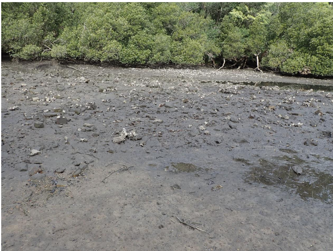
Figure 24 Beds of small rocks are present on both sides of the creek channel below the sandstone retaining wall
