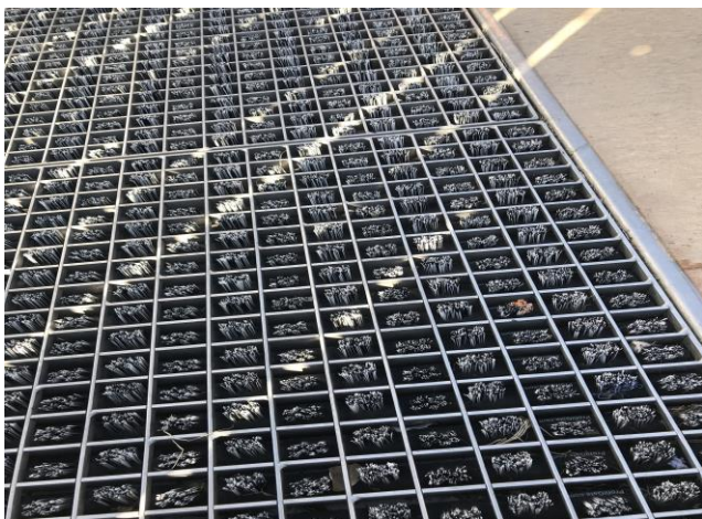
Photo 9: Containment strategy example 2: Pedestrian gate mats that capture the infill
