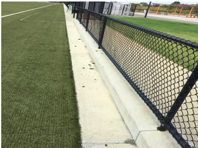
Photo 8: Containment strategy example 1: Curb to reduce the infill being dispersed outside of the field of play
