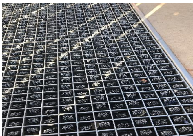
Photo 31: Pedestrian gate mats that capture the infill
