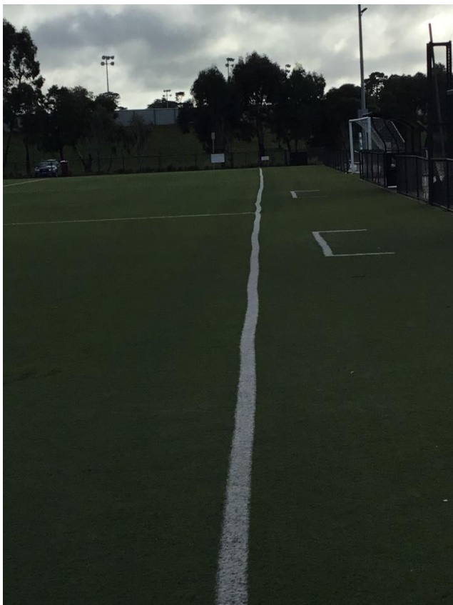
Photo 16: Line movement when there is not adequate infill and the cleaning machine goes over the lines it can stretch the surface
