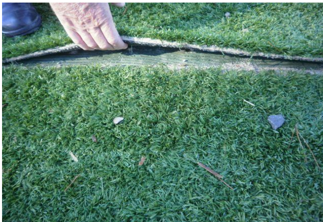
Photo 18: Seam has come apart, needs specialist to sew and or re-glue
