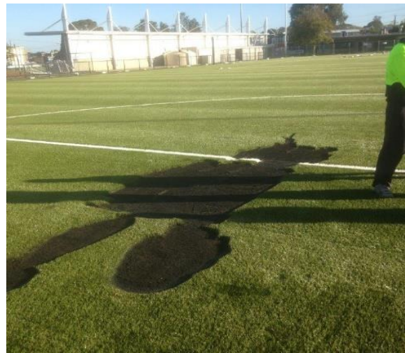
Photo 34: Vandalism can entail a whole section being cut out and replaced
