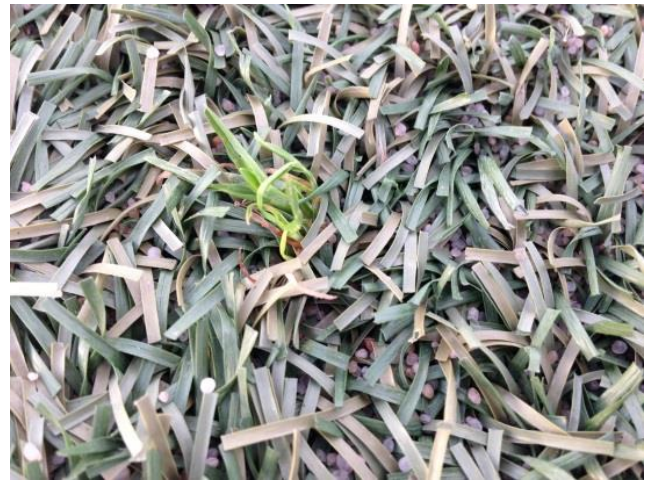
Photo 5: Turf not maintained adequately is showing the yarn is being bent over due to lack of infill and weeds are being allowed to grow
