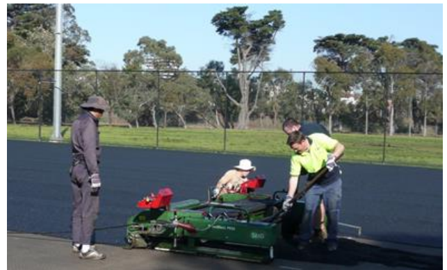
Photo 29: In-situ shockpad being laid (source: Polytan)
