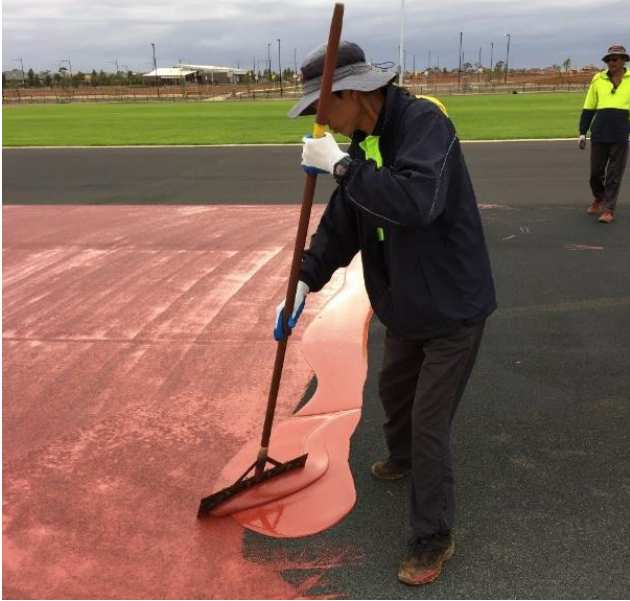
Photo 33: Application of wearing layer over rubber base mat
