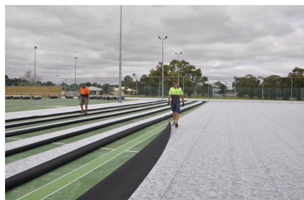
Photo 37: Installation of prefabricated mat system
