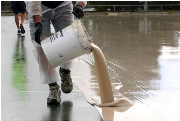
Photo 38: Application of gel system
