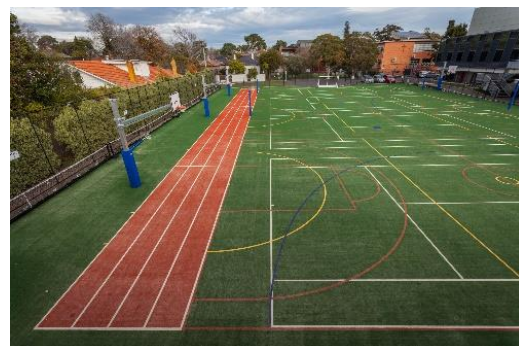
Photo 3: Multi-sports facility Ilim College, Vic (source: Grassports Australia)
