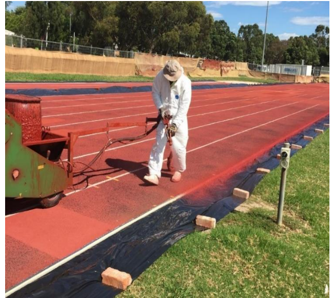
Photo 32: Application of spray coat
