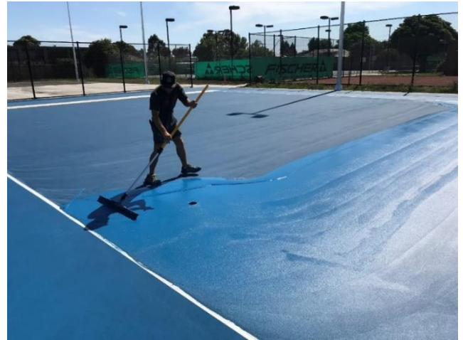
Photo 36: Application of acrylic system
