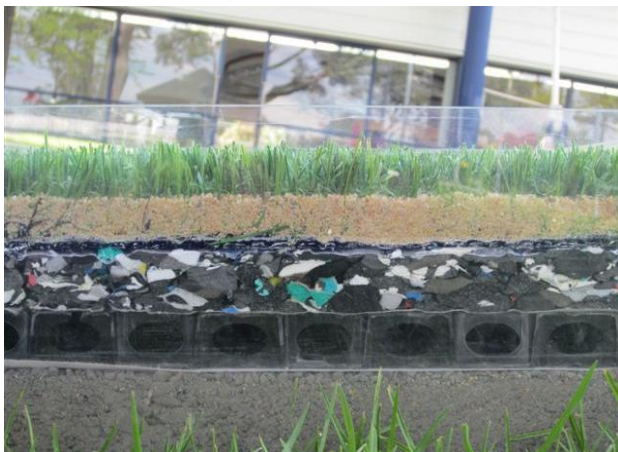
Photo 30: Example of horizontal drainage cell under shockpad (source: Wayne Stuart - City of Swan, WA)
