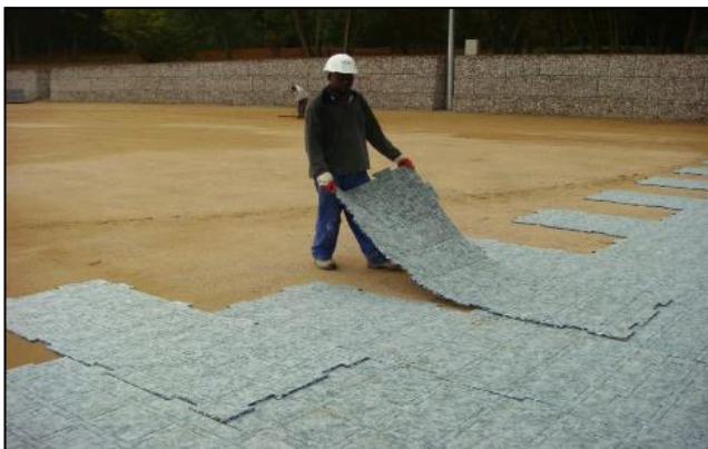
Photo 28: Prefabricated Shockpad being laid (source: Team Sports)
