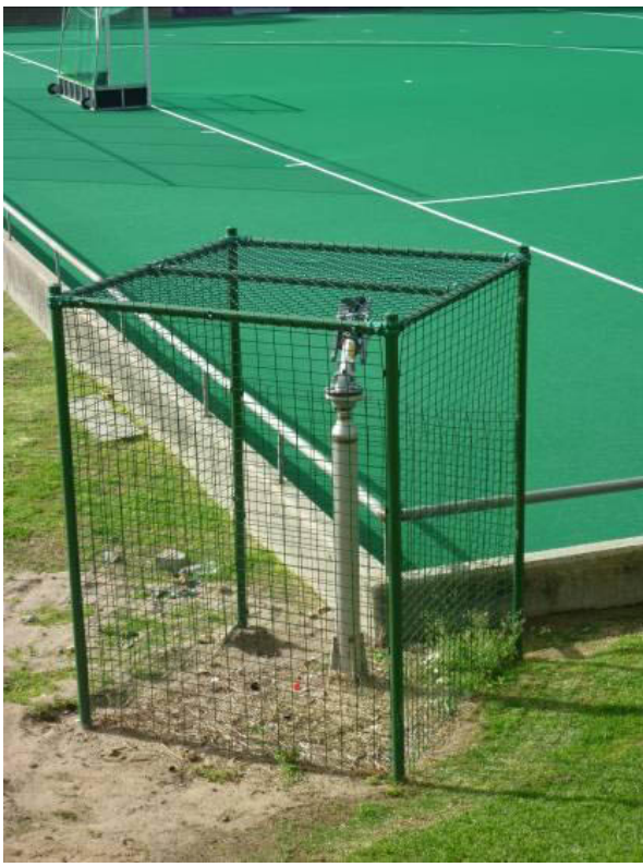
Figure 1: Water-based un-filled synthetic hockey pitch surface and irrigation point
