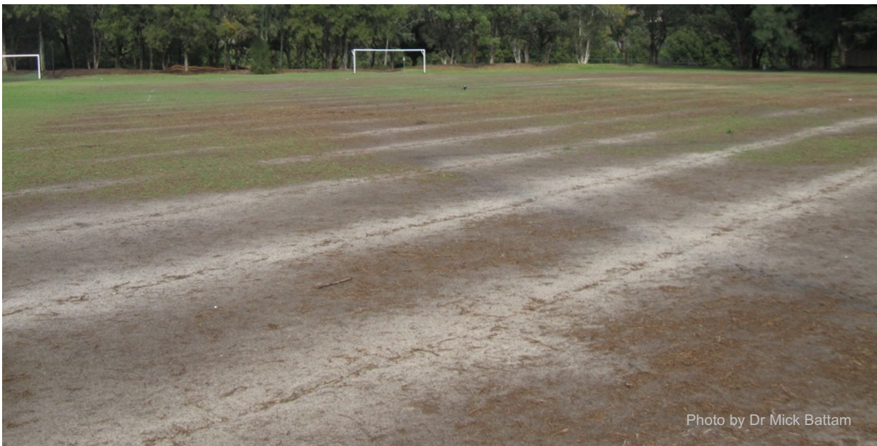
Figure 16.1: This field had slit drainage installed, enabling it to be used more often, but the turf cultivar could not handle it. As such, the field had to be reconstructed, with additional costs then needed to reinstate the drainage system. Install slit drainage after other works are complete.
