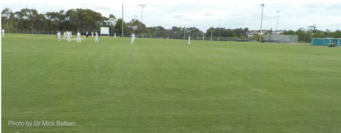
Figure 16.2: When Kahibah Oval was reconstructed the soil was fully amended and the new turf established from sprigs (upper) instead of laying sod. This was done due to budget limitations. With a slow draining base, and a turf wicket table, the site still requires a slit drainage system, which can be installed now that other works are complete. The new surface was fully covered in approximately 5 months, with soccer returning that winter and first grade cricket matches the following summer (lower).
