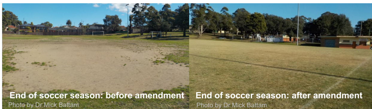
Figure 17.1: Incorrect field construction practices meant this field performed so poorly that it was reconstructed every 3 to 7 years. However, the soil was fully amended in 2017, with the turf now easily able to handle the sport usage levels.
