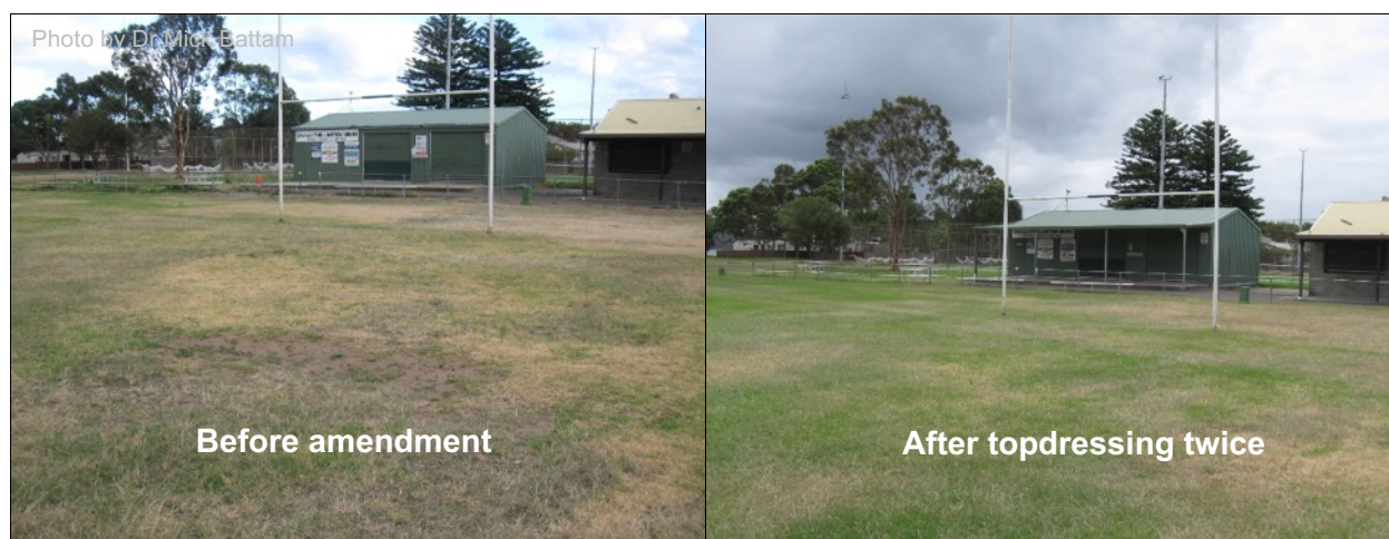
Figure 14.10: Parbury Oval at Swansea would ideally be reconstructed, but major improvements were achieved in the short term by topdressing with a suitable soil amender and aerating. Interim works such as these are often needed on fields that may not be reconstructed for several years.
