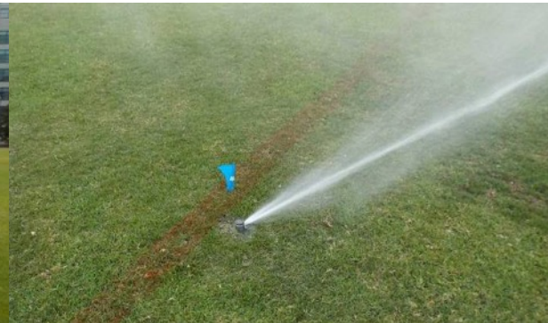
Examples of sprinklers leaking from riser seal or from below the sprinkler.
