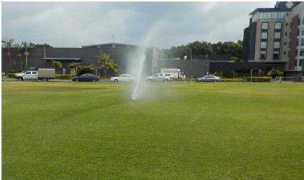
Examples of sprinklers leaking from riser seal or from below the sprinkler.
