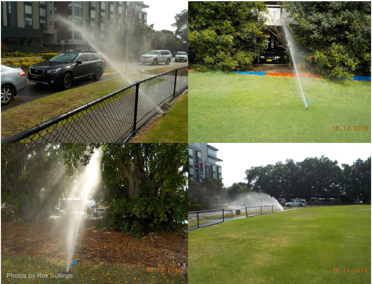
Heads with incorrectly adjusted arcs of coverage.
