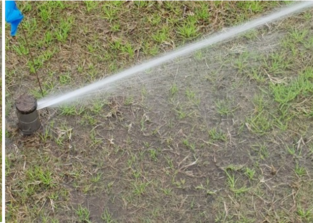
Examples of sprinklers leaking from riser seal or from below the sprinkler.
