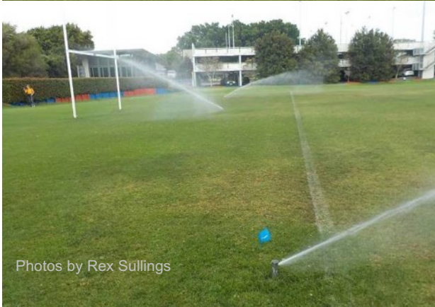
Heads with excessive misting
