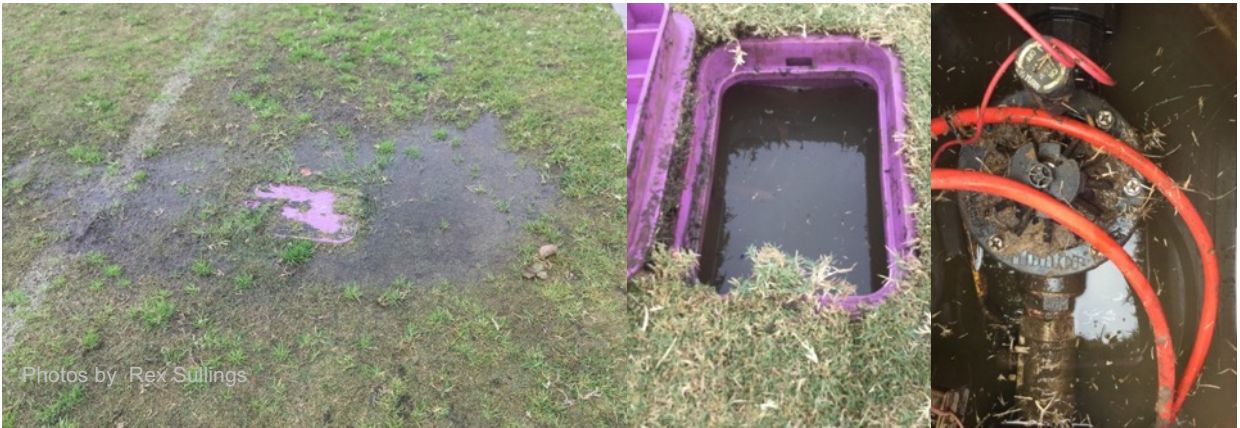
Examples of leaks at valves
