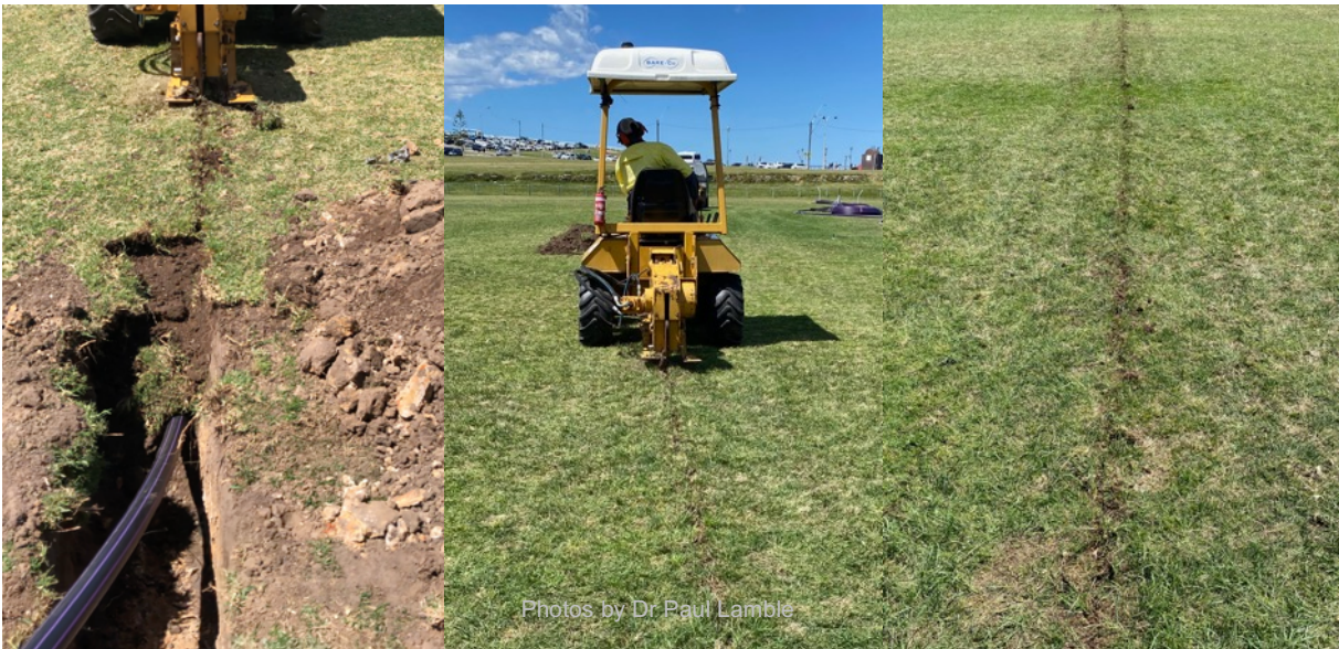
Figure 11.6: Installation of irrigation pipework using a plough
