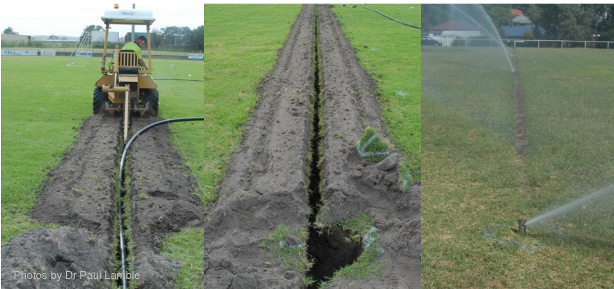
Figure 11.5: Installation of irrigation pipework using a chain trencher
