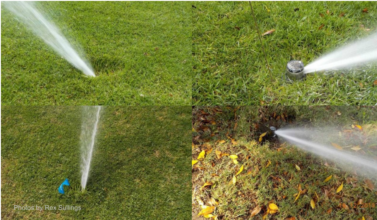
Heads that are too low (located well below grade)
