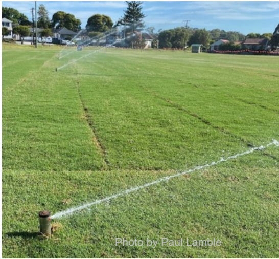
Low pressure (well below manufacturer's recommended minimum)
