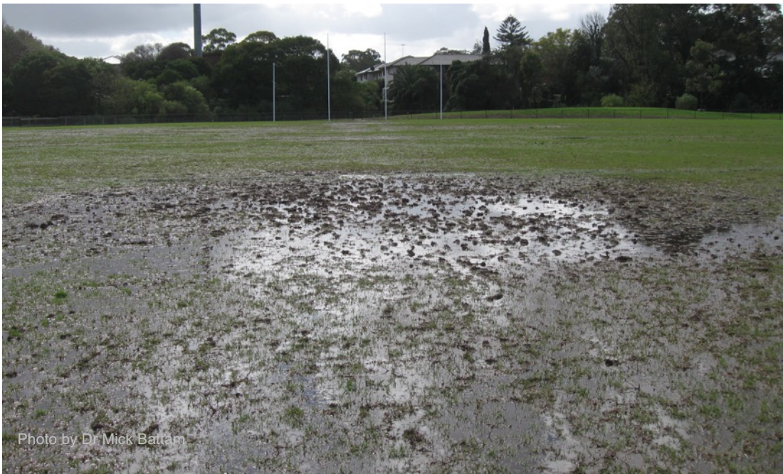
Figure 9.6: Field with a slit drainage system that was rendered useless by topdressing with 80:20. Whilst this material is very sandy, it has an infiltration rate much lower than the sand used in the slit drains.
