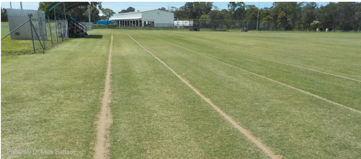
Figure 9.2 Recently installed slit drainage system showing the sand extending all the way to the surface. The turf will grow across the slits from the adjacent areas, so they are less visible over time.
