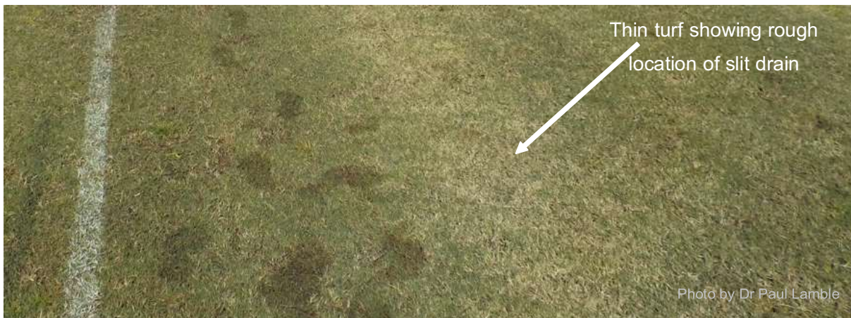
Figure A.2: Saturated areas between sand slits that won't drain due to soil issues that were not addressed.
