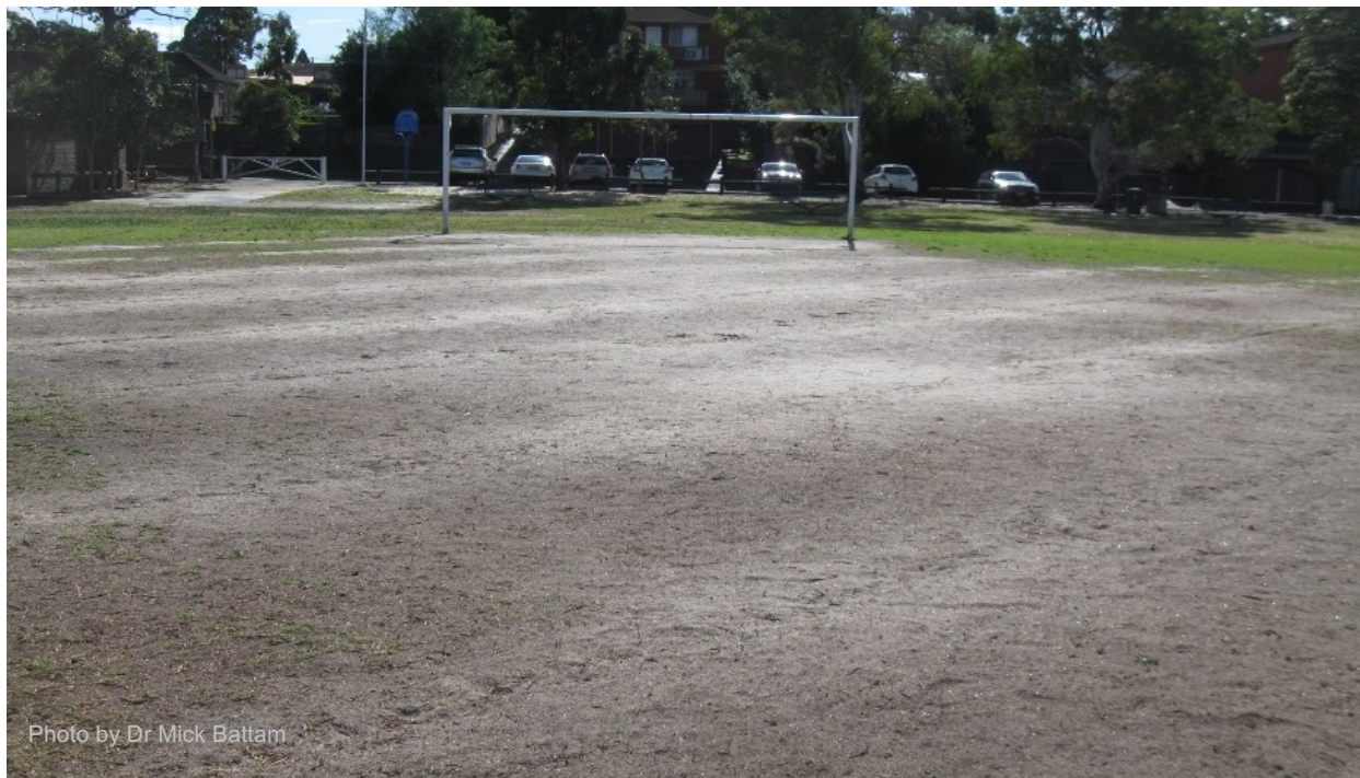
Figure 9.4: Slit drainage was installed in this field enabling it to be used more often, but the turf cultivar could not handle the wear. As such, the field had to be reconstructed, with additional costs then needed to reinstate the drainage system. Install slit drainage after other works are complete and an acceptable playing surface can be maintained.
