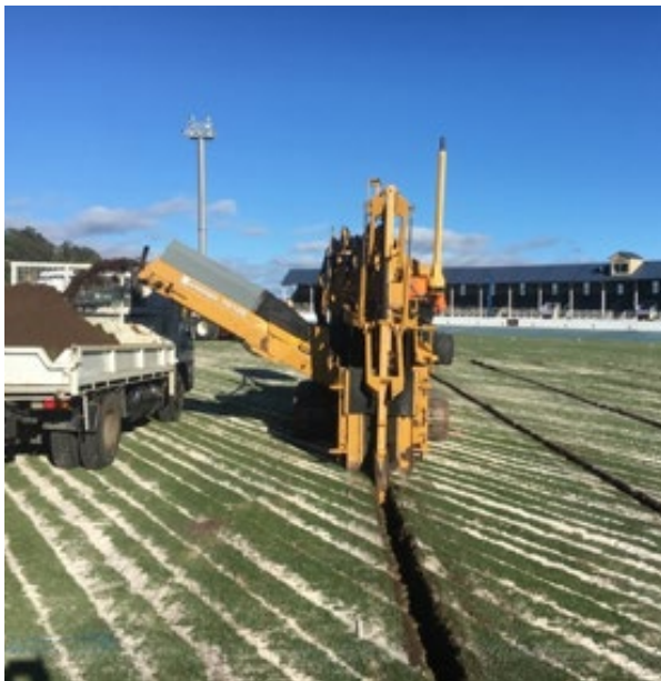
Installing sand slit drains into existing sportsfield
