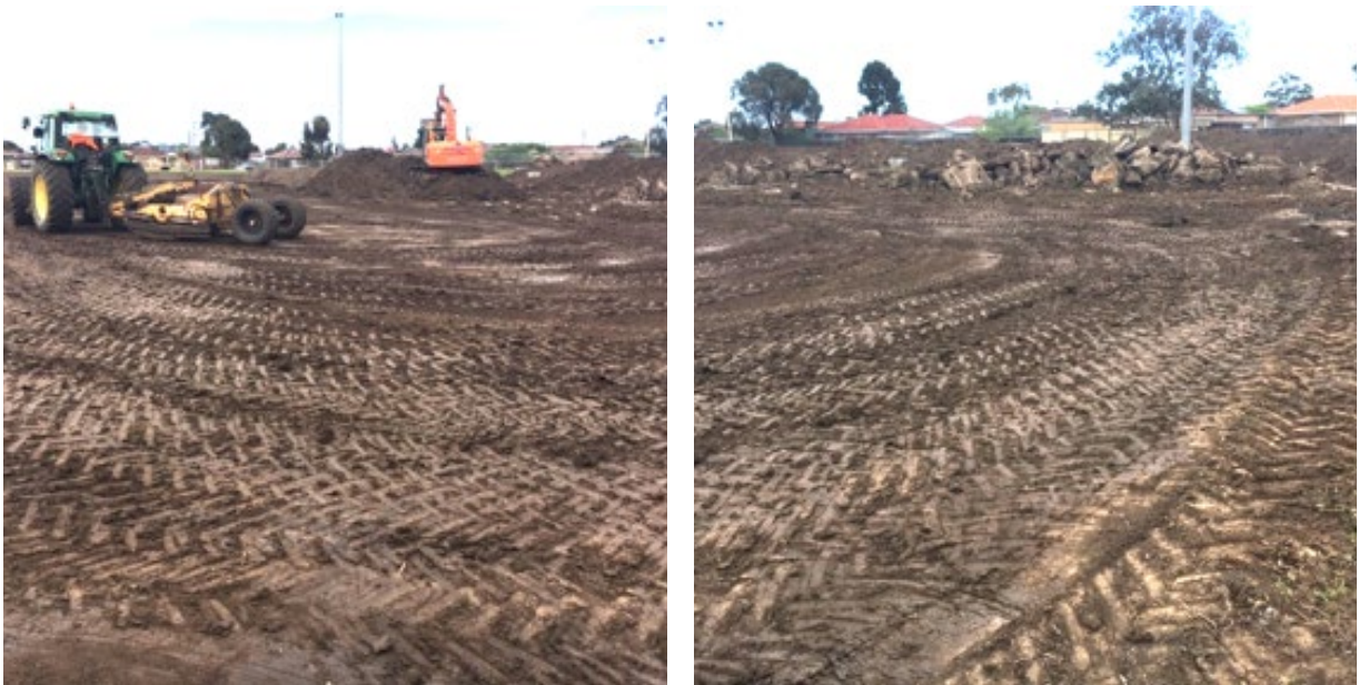
Subgrade work on a sportsfield
