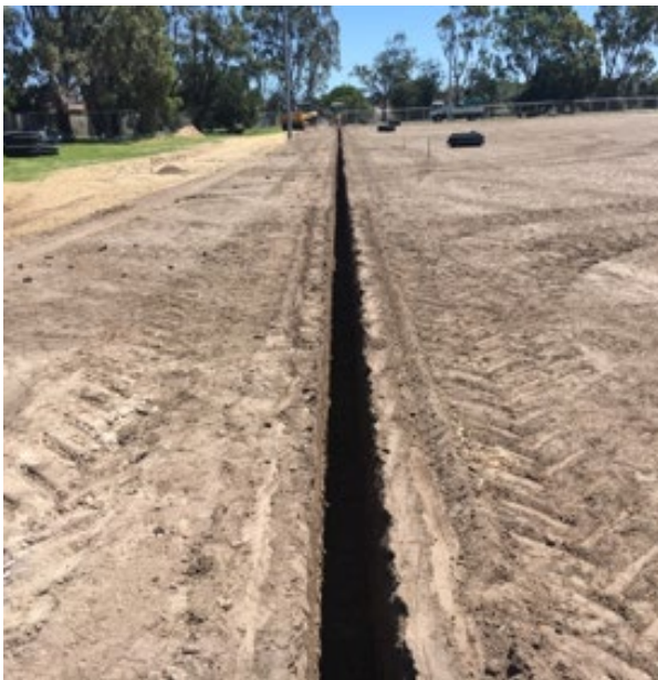
Trench dug prior to installing drain
