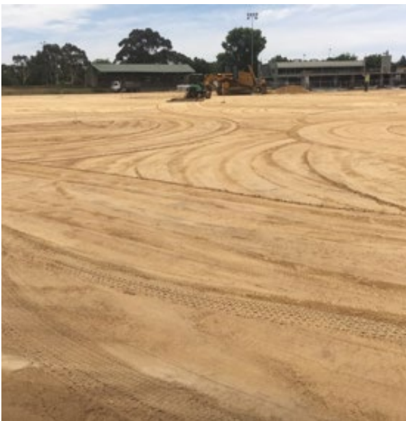
Installation of sand root zone layer
