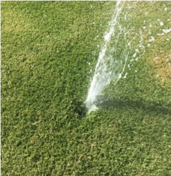
Low sprinkler head
