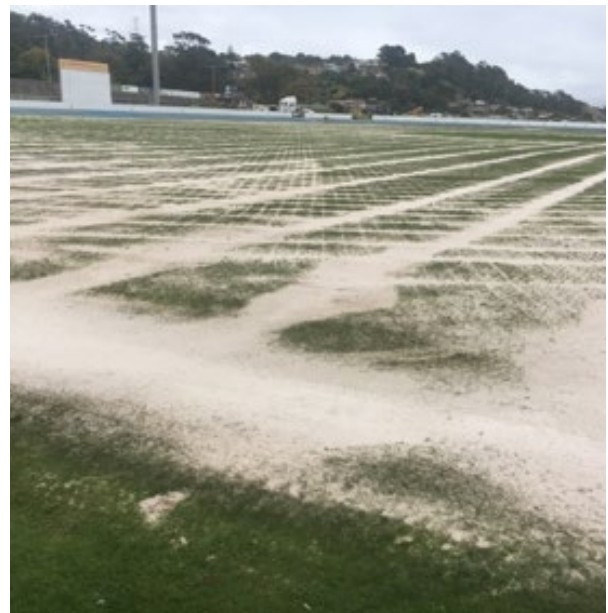
Installing sand slit drains into existing sportsfield
