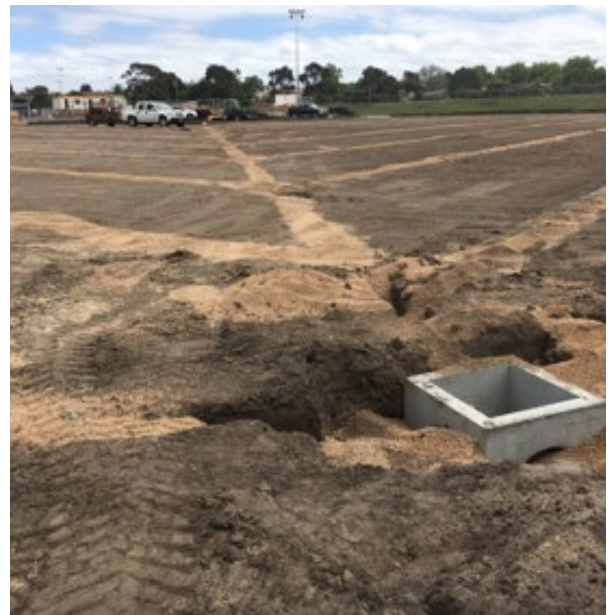
Subsurface drainage being installed in oval
