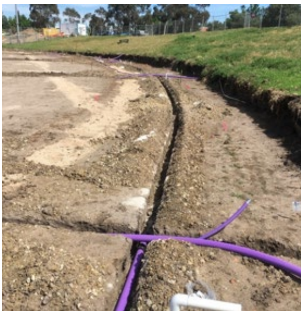
Installation of irrigation pipework
