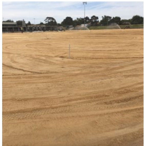
Installation of sand root zone layer
